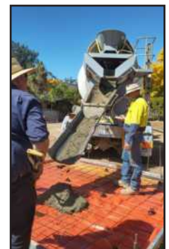
Preparing and pouring the cement for the Layer facility
