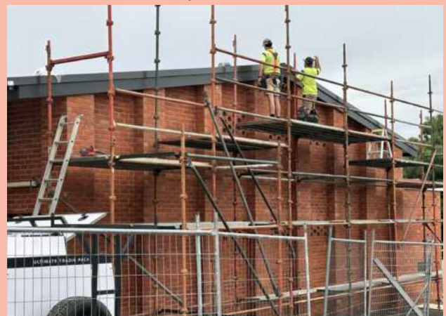
Finishing touches to new roof and eaves
